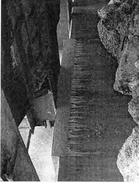
e. Completed interior girder seat
