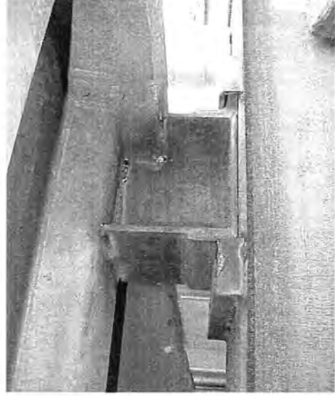
d. Exterior girder support in place at the north abutment
