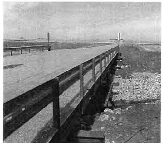
b. Installation of the thrie beam
