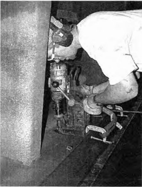
a. Drilling holes for the transverse threaded rod
