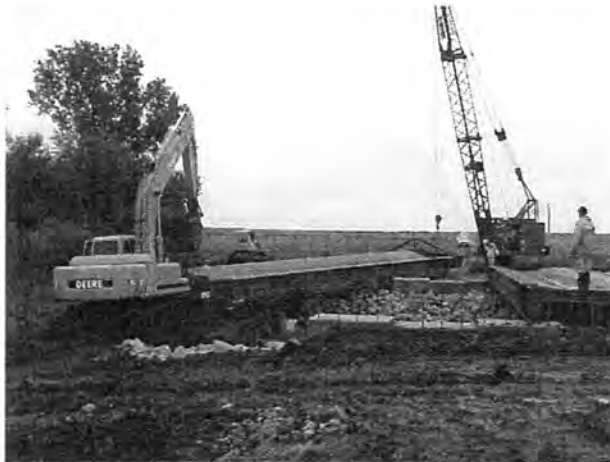
b. Flatcar placement on the cap beams
