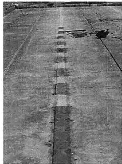
d. Top connection plates after concrete placement
