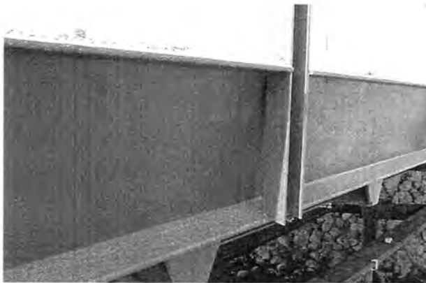
a. Addition of guardrail posts
