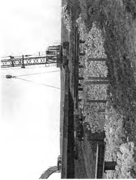
b. Placement of the 89-ft RRFCs
