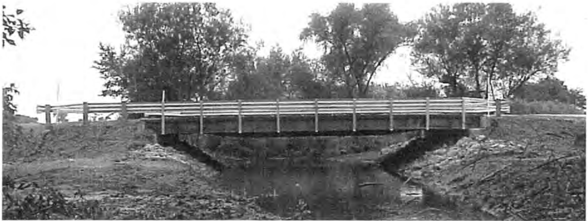
Figure 3.7. Finished Buchanan County RRFC Bridge.
