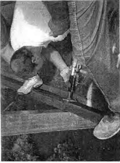
b. Nailing on the side rail for the driving surface
