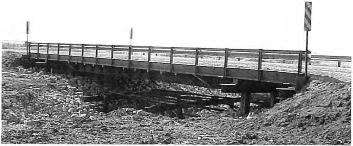
Figure 3.15. Finished Winnebago County RRFC Bridge.
